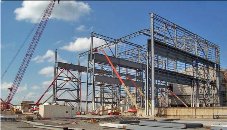
Gerdau Ameristeel - Melt Shop Reheat Furnace Building Jacksonville, Florida
